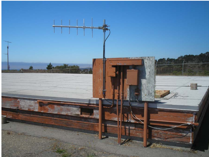
Figure 4-3: Reservoir and Telemetry
