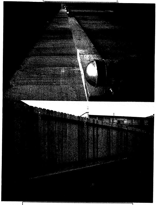
OUR (8") THICK CONCRETE RETAINING WALLS, W/GALV. POSTS INSERTED/CAPPED. NO TERMITES/RUST/GROUND CONTACT #2 AND BETTER SELECT, TIGHT-KNOT WESTERN RED CEDAR, W/DOG EARS
