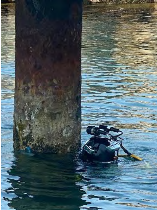
Figure 1: HOI Diver Inspecting Rincon Island Piles
