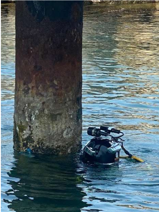
Figure 1: HOI Diver Inspecting Rincon Island Piles
