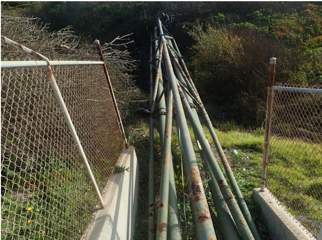
Another view from the north side and above.
