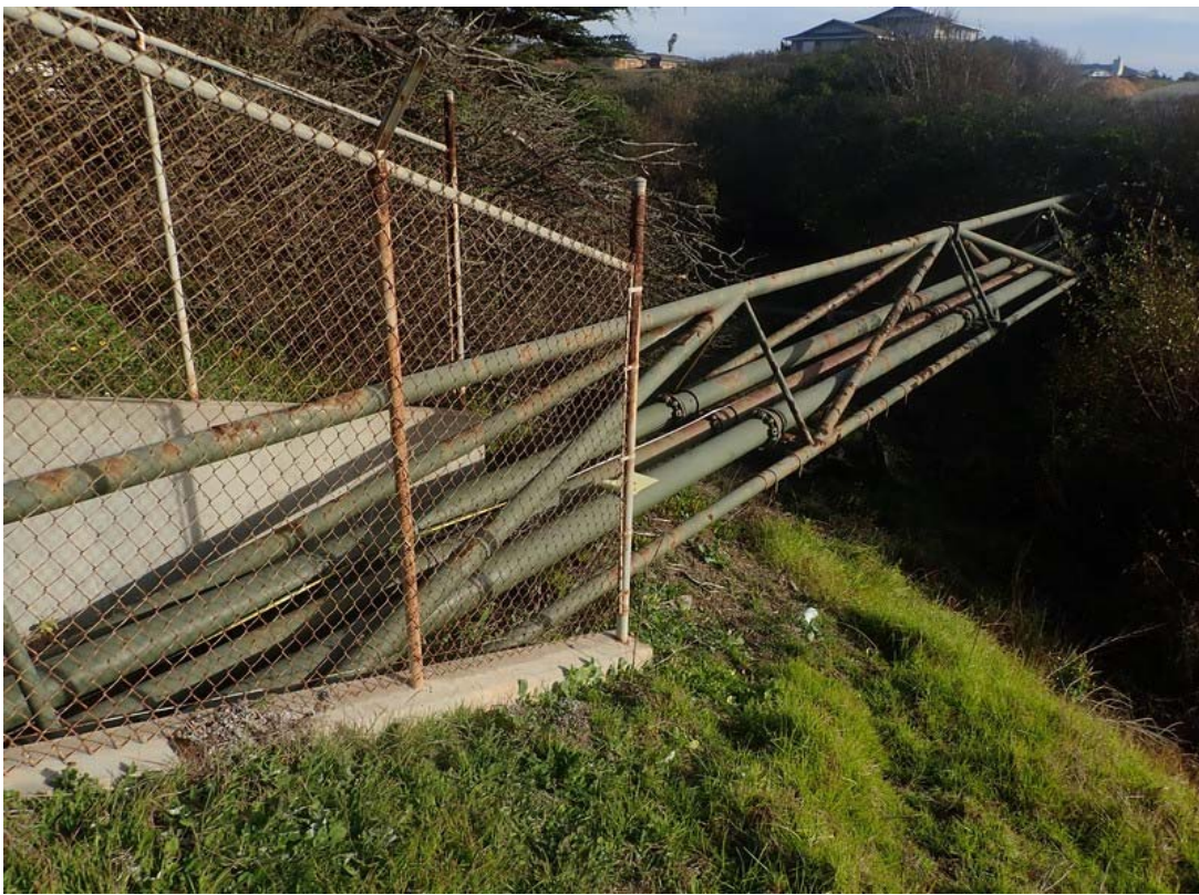
Bridge overall view from the north side.
